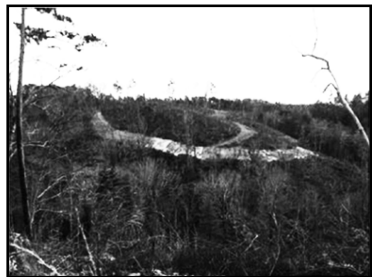
After: Following three years of monitoring the site and highlighting the negative effects of logging, the Forest Service admits failure and begins expensive re-mitigation of the site with recontouring, reseeding, and adding a mulch mat. The new ranger has cleaned house and begun new practices to make sure this doesn't happen again.
