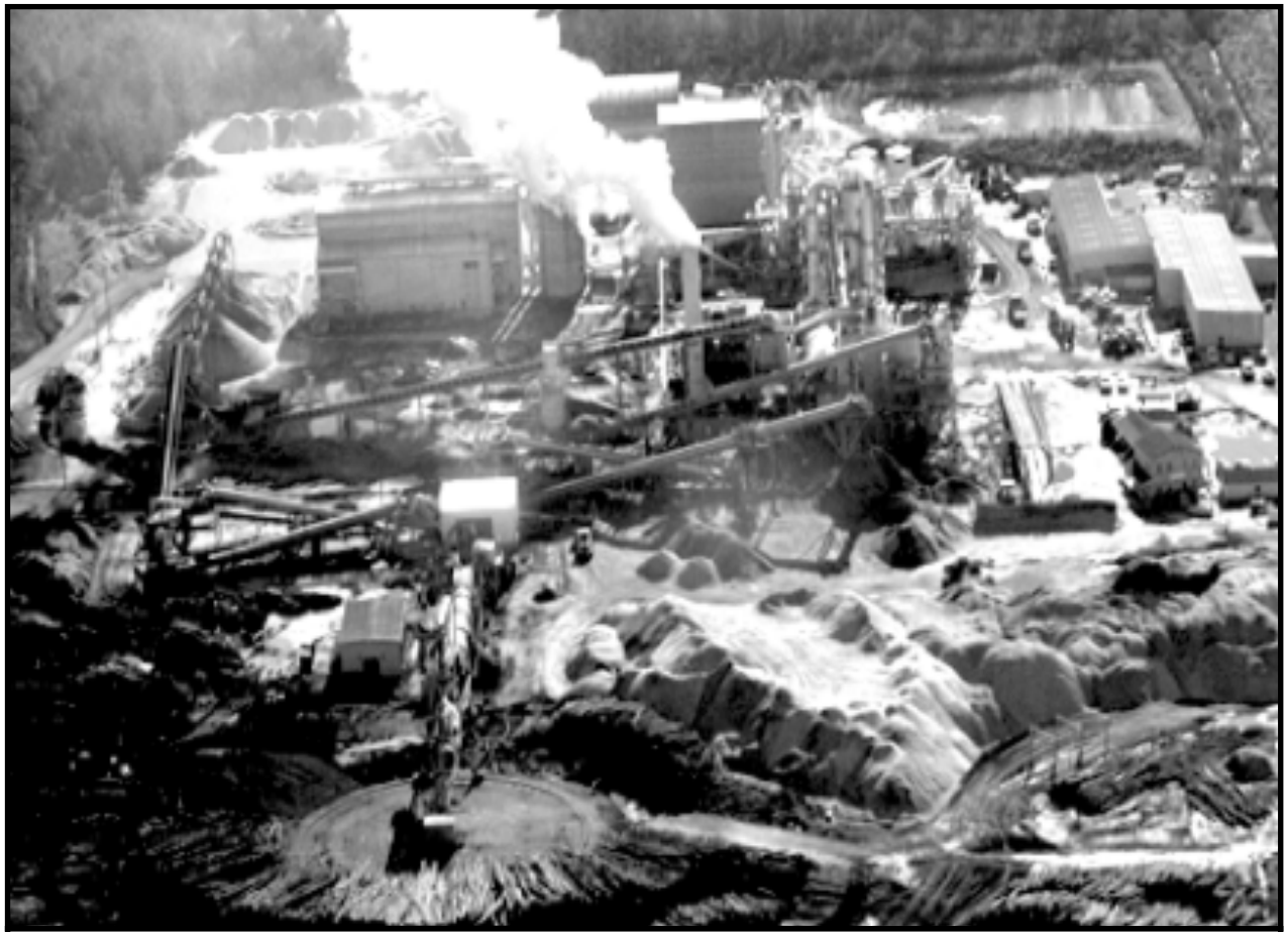
Overhead shot of the Enviva Ahoskie Facility
