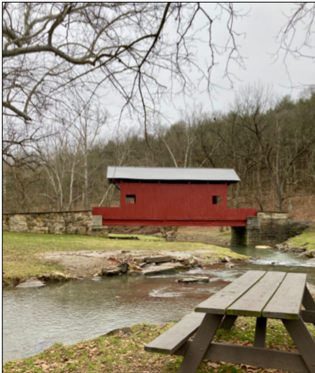
One of two covered bridges in Mingo Creek Park. Photo by Kara Kukovich.
