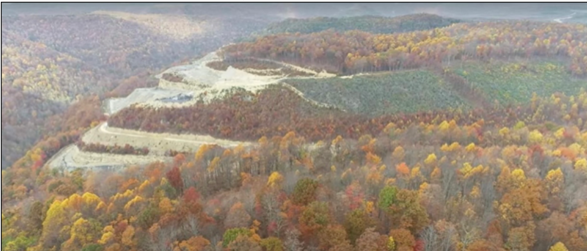
Bottom photo: Lexington Coal Company's Crescent #2 mountaintop removal permit, renewed by WVDEP on Jan. 12 in spite of serious violations and unpaid fines. Photo by CRMW/Junior Walk.
