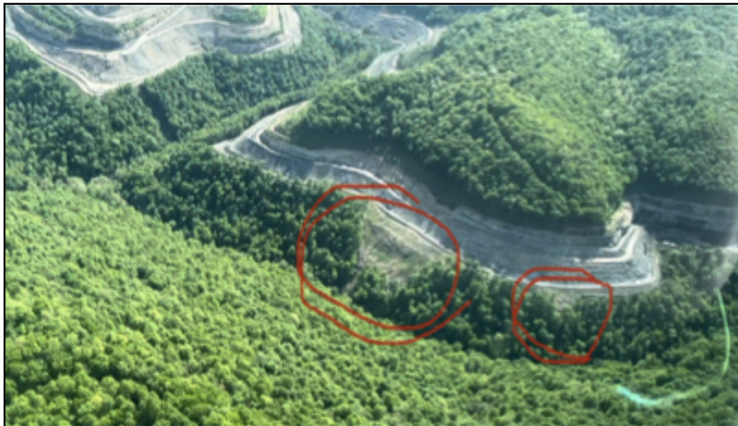
Above: Flyovers reveal two potential violations of sediment control or downslope spoil requirements at the edge of Lexington Coal Company's Crescent #2. Photo by Vernon Haltom, CRMW. Flight courtesy of SouthWings Volunteer Pilot Scott Simonton.
