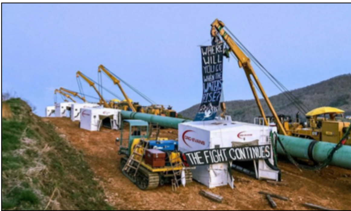
photo by Appalachians Against Pipelines.
