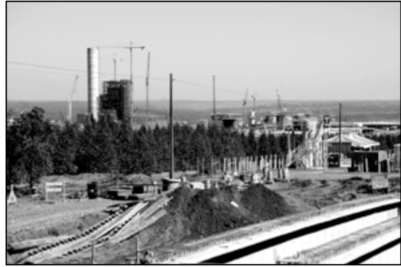
Construction site of the world's largest pulp and paper mill.
