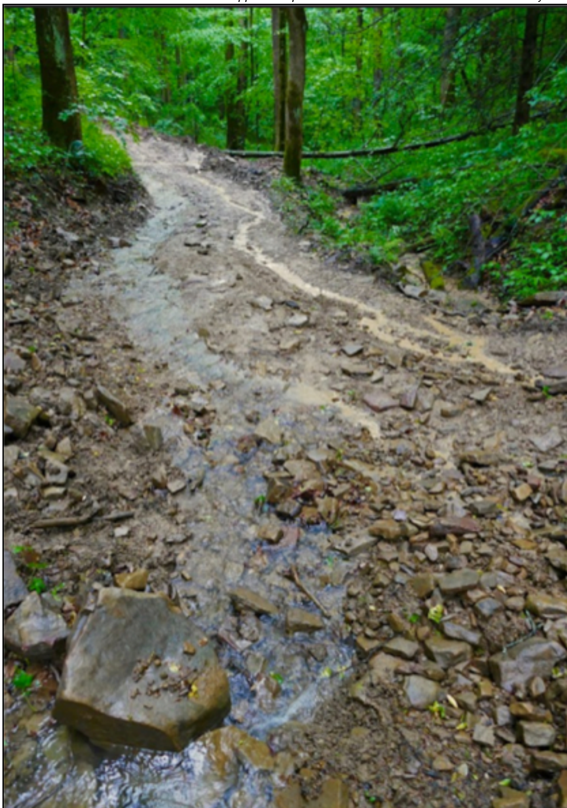
A poorly maintained trail for motor vehicles erodes sediment into the Upper Camp Branch near Breaks Interstate Park. Photo by TCC
